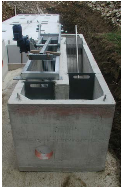
Figure 1: Screening plant
