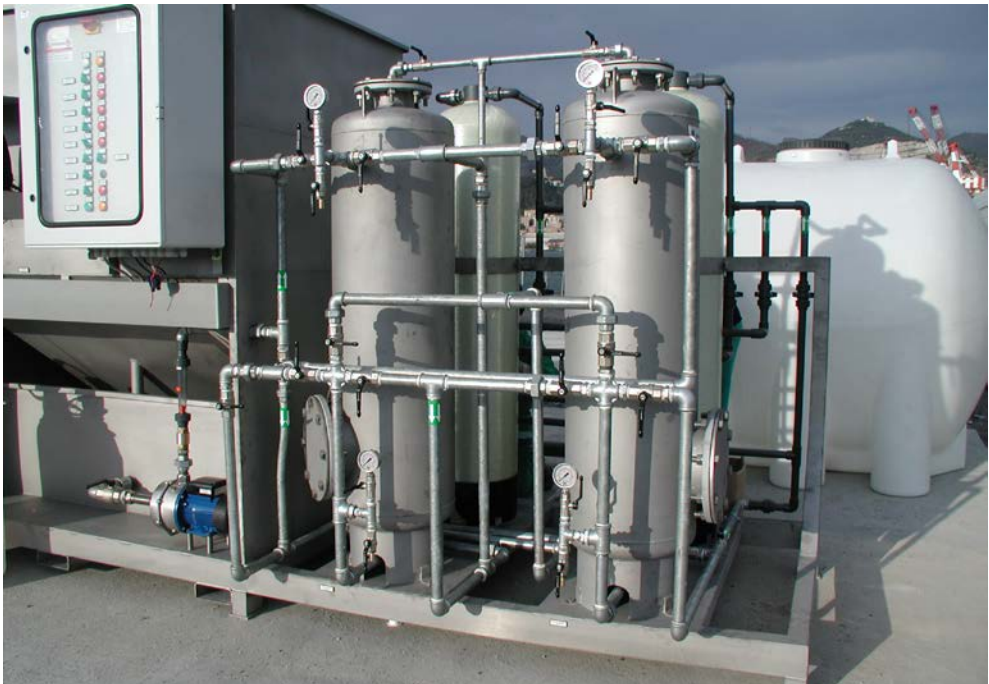
Figure 6: Clariflocculation plant with final filtration
