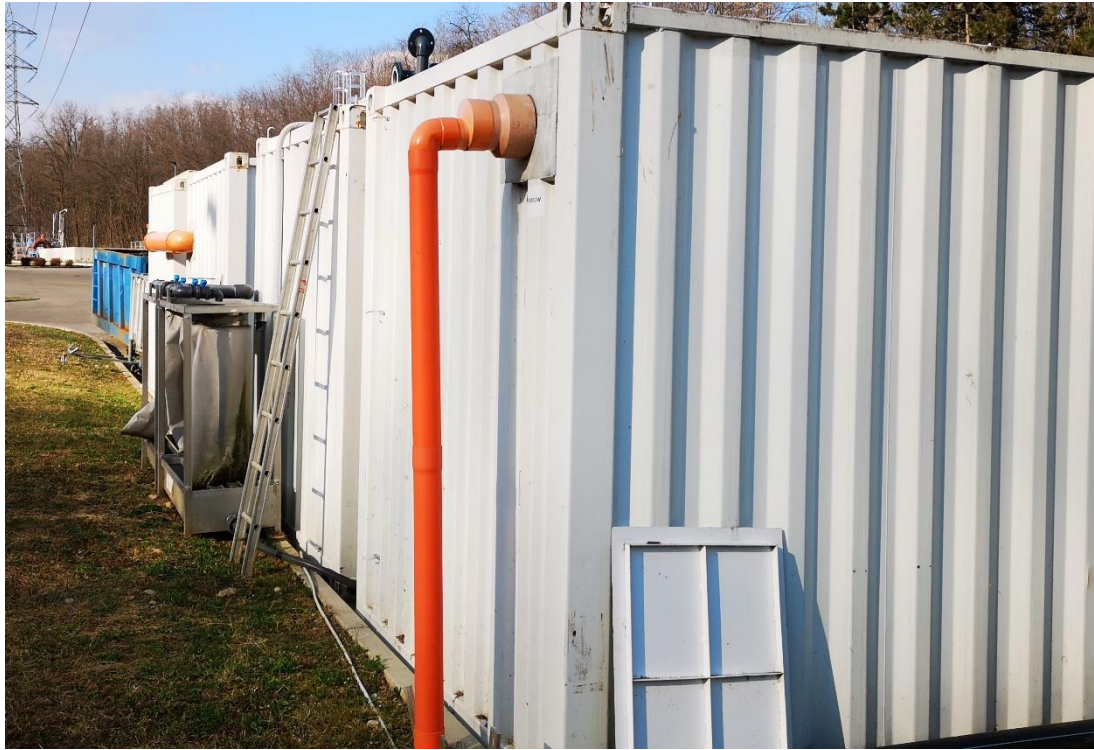
GREEN MBR system Civil Waste Water Treatment Plant Containerized
