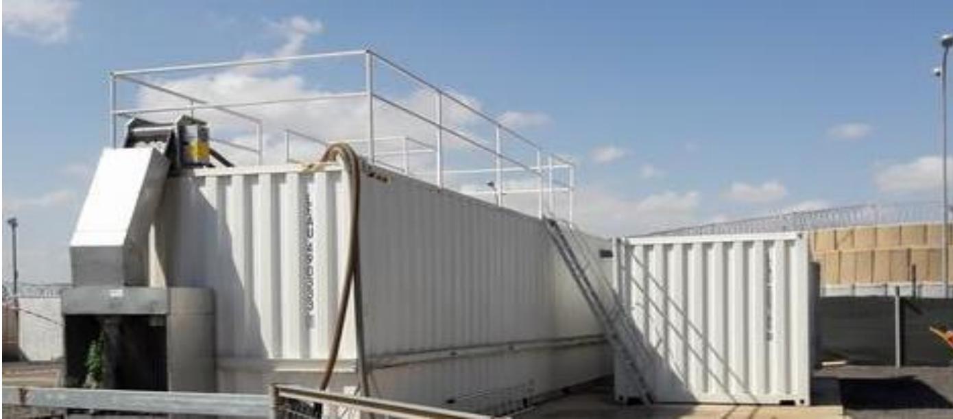
MBBR system Civil Waste Water Treatment Plant Containerized
