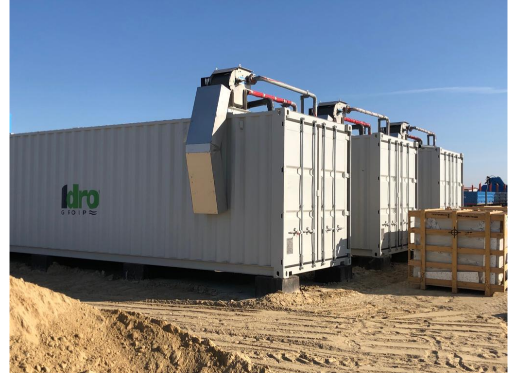
MBR system Civil Waste Water Treatment Plant Containerized In 40' insulated Containers
