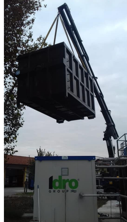
MBR system Civil Waste Water Treatment Plant Containerized
