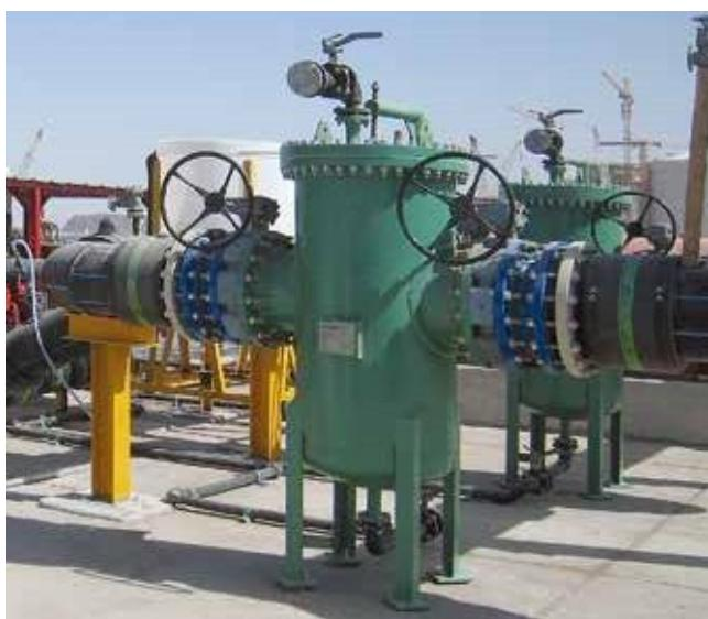
View of filtration system with valves.
