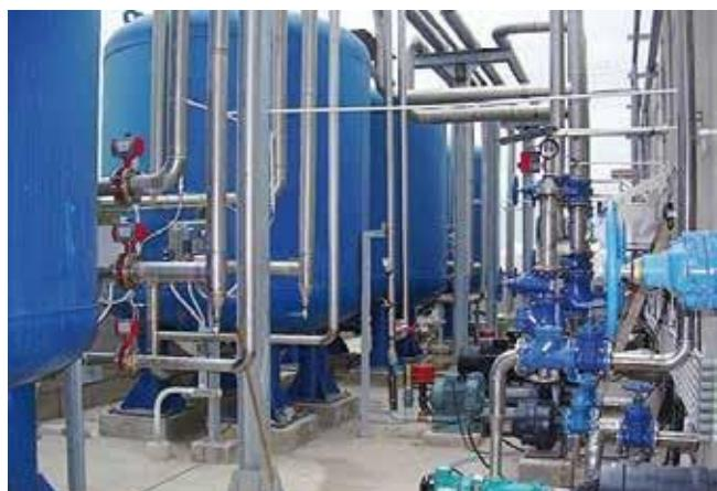
Quartz filtration unit for suspended solids removal
